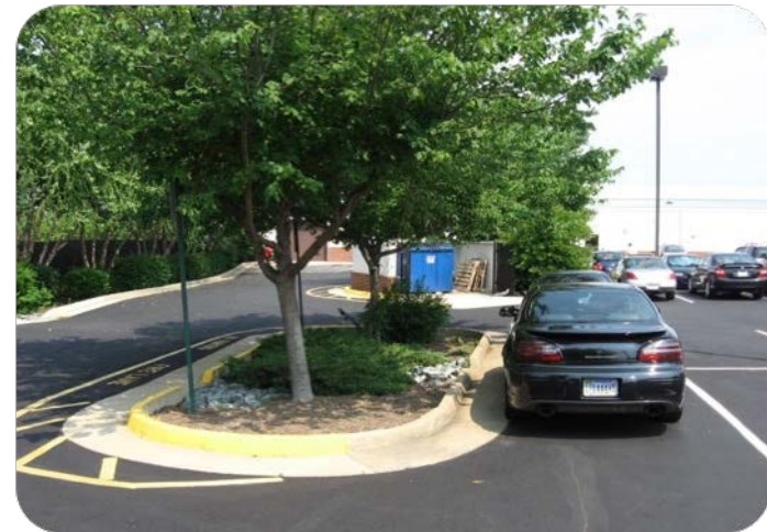
Parking lot infiltration, Stafford County, VA
