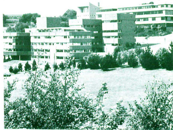
Exeter University Campus; Law School Building in foreground
